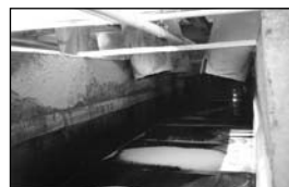
Photo D: After each 24' section was put in place they were field welded into a single 96' long seamless unit. Minimal fasteners (only 24 in the first section) and leading edge protectors complete the installation.
